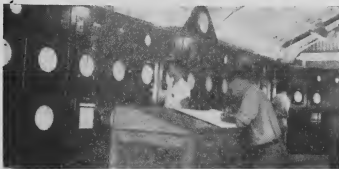
Above, each of the new aviation-gasoline facilities has a panel board, its "nerve center", like this control room at the new Alkylation Plant. Here operating conditions from all parts of the unit are revealed and recorded. Below, one of many unusual features of the new "Cut" Plant is the elevator at left, needed because of the great height of the structure, 235 feet, or equal to a 20-story building. This enormous equipment (see picture on page 1) is so much controlled by automatic devices that only eight men are required for its operation. Top page 7, this new compression plant handles 35 million cubic feet of various refinery gases per day, which then go to the Gas Absorption Plant for recovery of light ends. Bottom, page 7, the tower of the new Alkylation Plant, a potent part of the new facilities, presents a striking design when pictured from an unusual angle.
